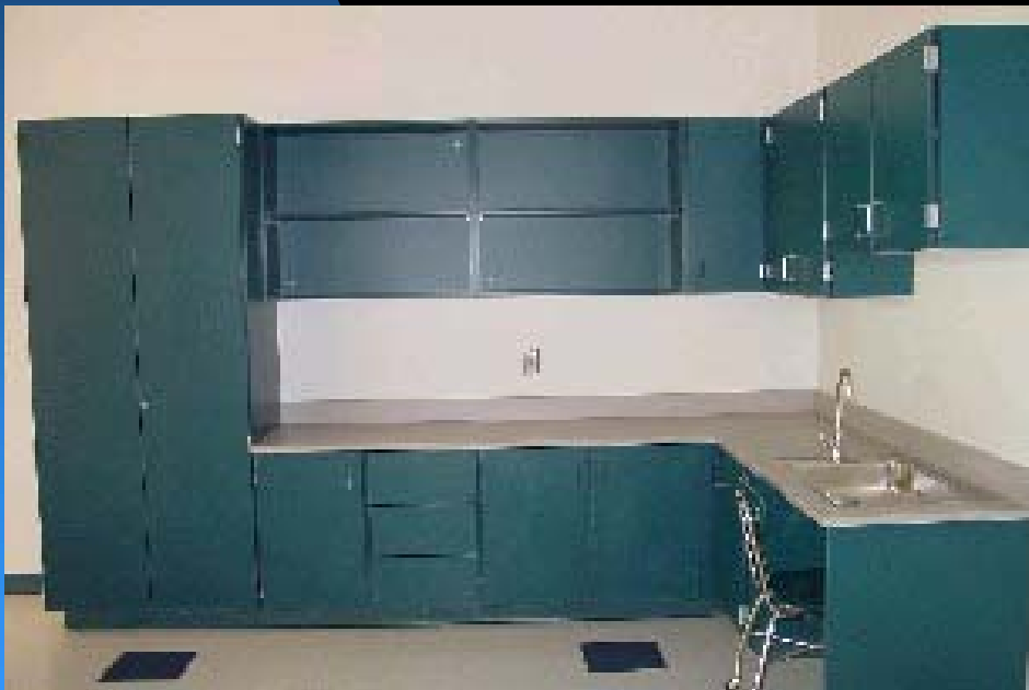
Example of Strawboard-Core Cabinets
