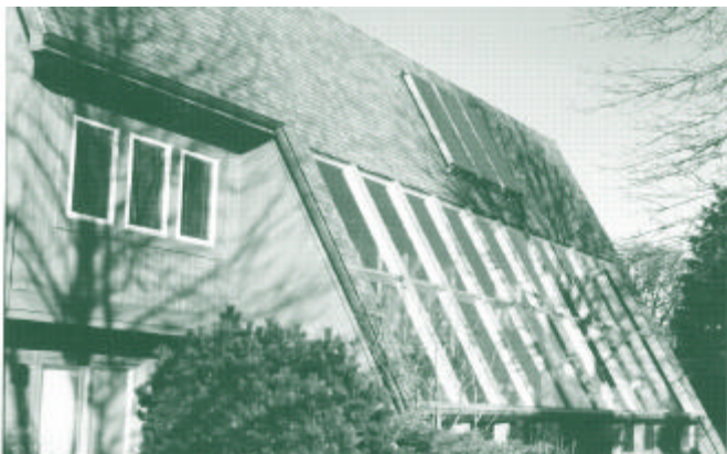
Solar thermal collectors (top) resemble the skylights on this Ohio home.
